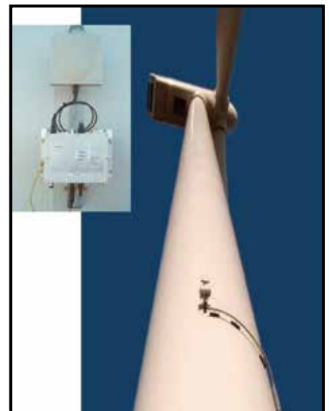
Wireless installation on tower.
