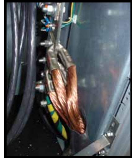
Figure 1. Termination for parallel ground connections on drive.
