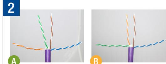
After cable is fully prepped, align your pairs in a 2 up, 2 down formation
