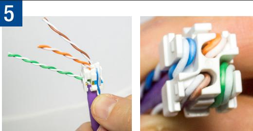
Untwist pairs (do not separate) just enough for the white conductor to reside on the outside. Bend all four pairs over and down the manager and lock into their respective channels.
