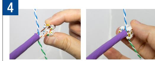
As you slide the cable manager down the wires, follow the printed arrows to turn the manager *clockwise* until the outer pairs can reside in between the outer channels. Cable manager should sit snugly on cable
