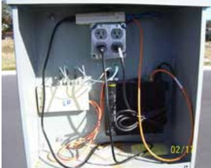
Magnum 6K Switch in typical lightpole installation
