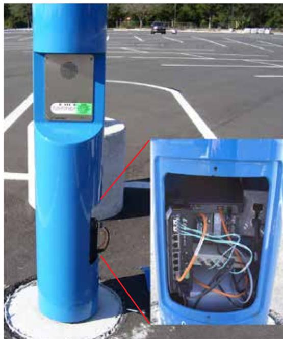
Magnum 6K Switch in typical Code Blue tower installation
