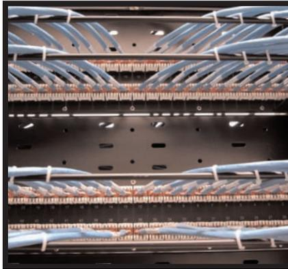
The blue-jacketed cables shown here are terminated to Belden IBDN GigaFlex Patch Panels in one of building's 13 IDF rooms. The Belden patch panels are built on patented technology designed to deliver exceptionally stable signal transmission performance.
