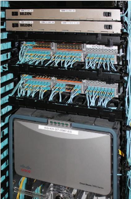
Designed using the latest switch fabric topology, the data center for MaineGeneral features two Cisco Nexus series 7010 core switches to distribute fiber to pods via Belden’s FiberExpress Ultra High-Density (UHD) rack-mount fiber connectivity system.
