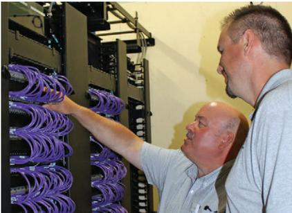
Built based on a mock TR evaluated during the IPD planning stages, Hallee (left) and Whitaker with E.S. Boulos deployed 1U blank panels above and below 48-port patch panels for each horizontal switch and used one-foot patch cords for aesthetics and manageability.
