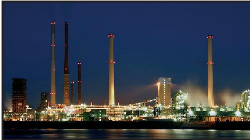
Here, the Schwelgern GmbH coking company belonging to the ThyssenKrupp Steel AG produces an annual 2.5 million tons of coke from coal for the neighboring large blast furnaces. The transformation takes place in a total of 140 of the world's largest coke furnaces
