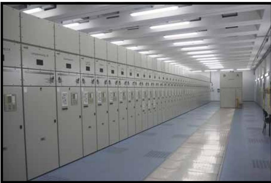
Protection and control level in a digital substation. Ethernet switches are inside the cabinets and allow communication among the different intelligent electronic devices (IEDs) in the station bus.
