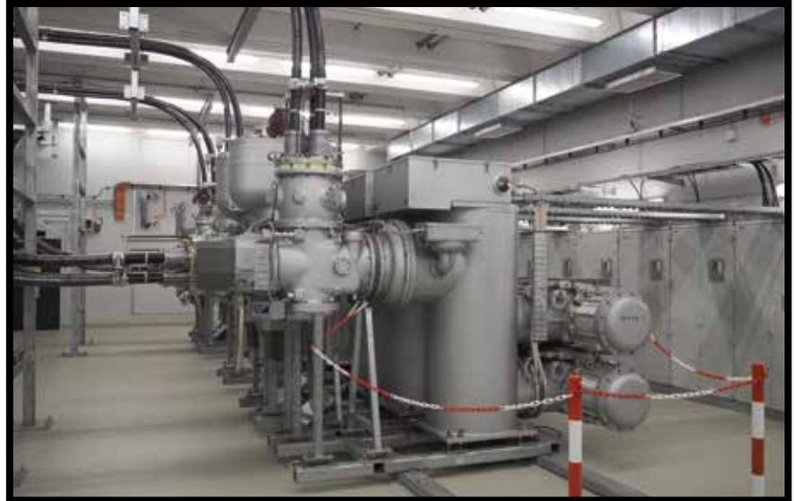
Gas-insulated switchgear (GIS) and bay control units in a substation.
